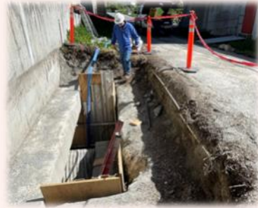
Excavation of expansion joint (left) and close-up view of buried expansion joint
